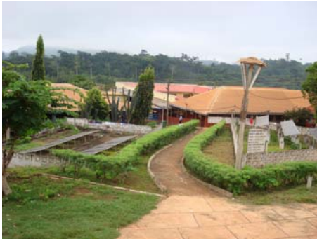
HOSPITAL WITH SOLAR PANELS ON LEFT
