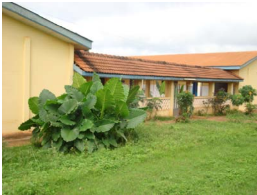
A new Isolation Unit for 32 beds Donated by a Charity based in Spain now lying idle following changes by Government. MOTEC has an eye on this structure.
